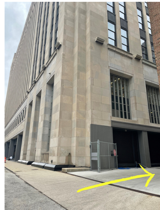
Entrance to access parking garage
