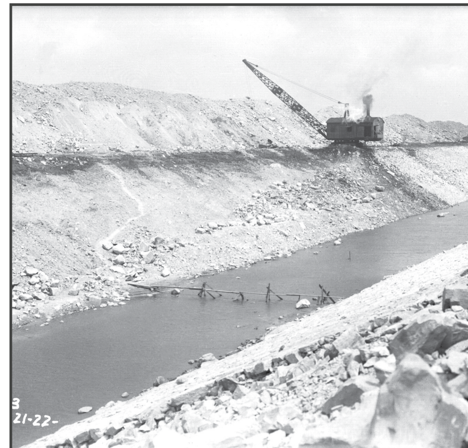
FIGURE 2: BUILDING THE CAL-SAG CANAL | Source: MWRD
