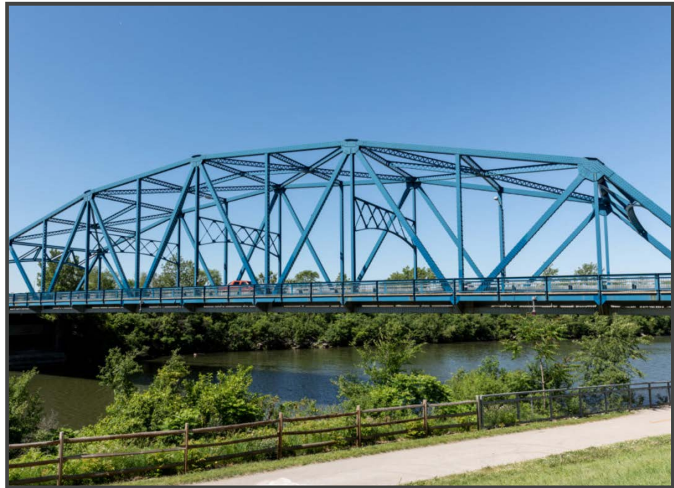
FIGURE 5: BRIDGE OVER THE CAL-SAG CANAL | Source: @Properties
