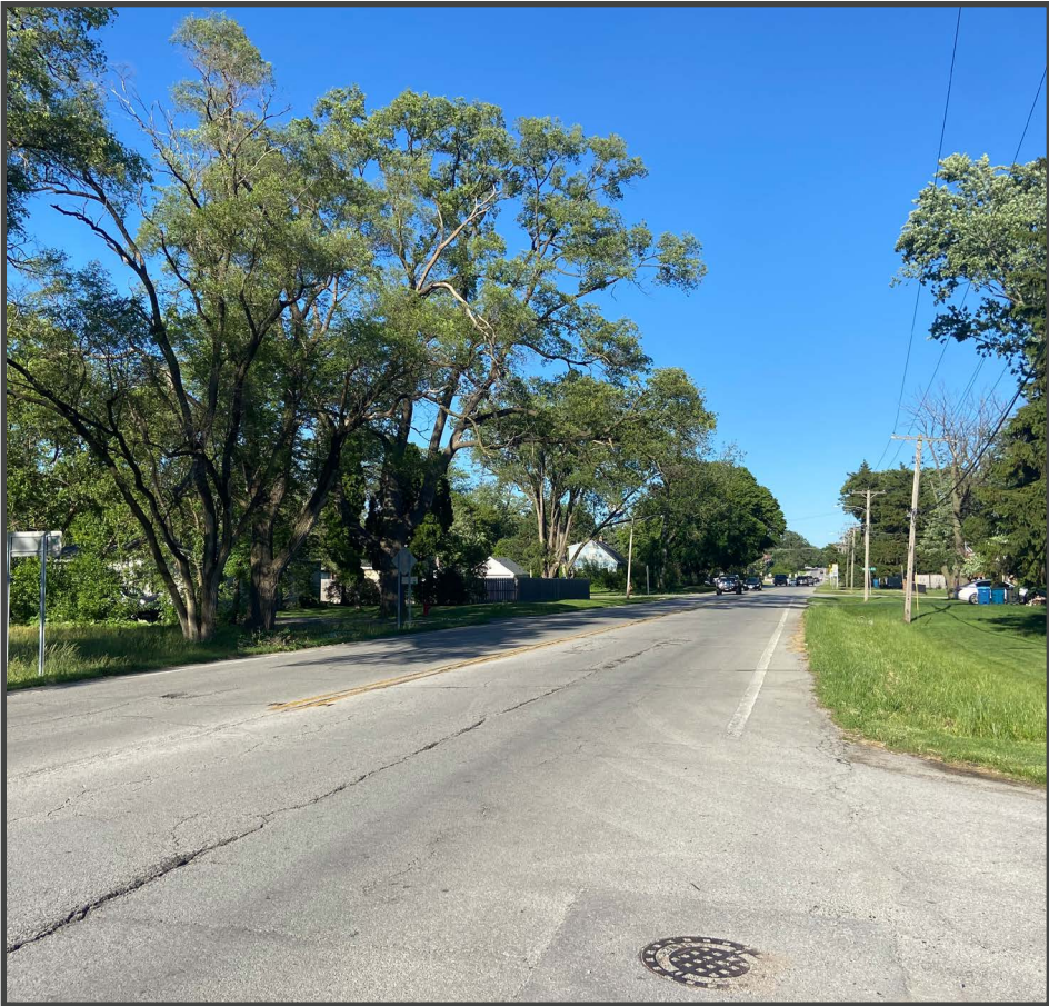
FIGURE 40: LACK OF SIDEWALKS ON 119TH STREET | Source: Epstein
