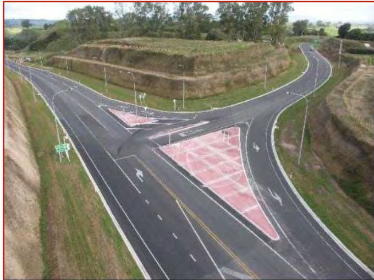
Figure 4-40. Example of a Realigned Skewed Intersection
