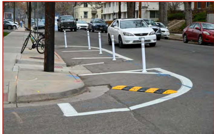
Figure 4-1. Paint and Post Curb Extensions
