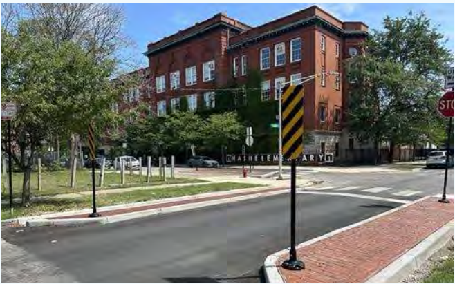
Bump-outs located at the intersection of Erie St and Lamont Ave at the northwest corner of Nash Elementary School’s campus shorten the crossing distance for students walking to school.
