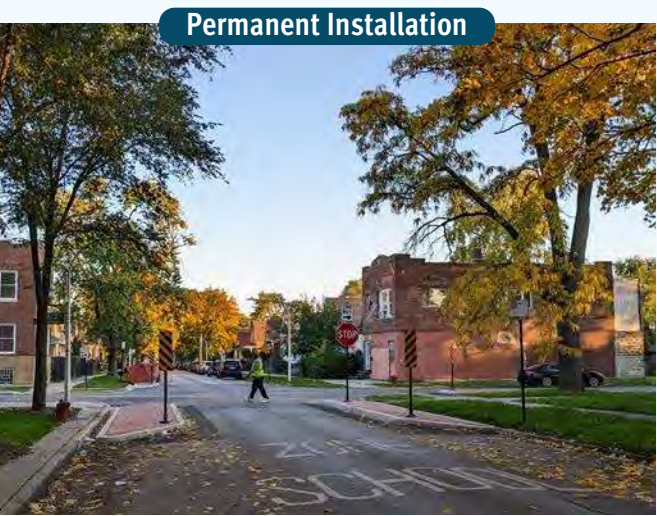
Rapid delivery bump-outs at intersections surrounding Lindblom Math and Science Academy were upgraded to concrete. These bump-outs slow traffic and improve pedestrian visibility.
