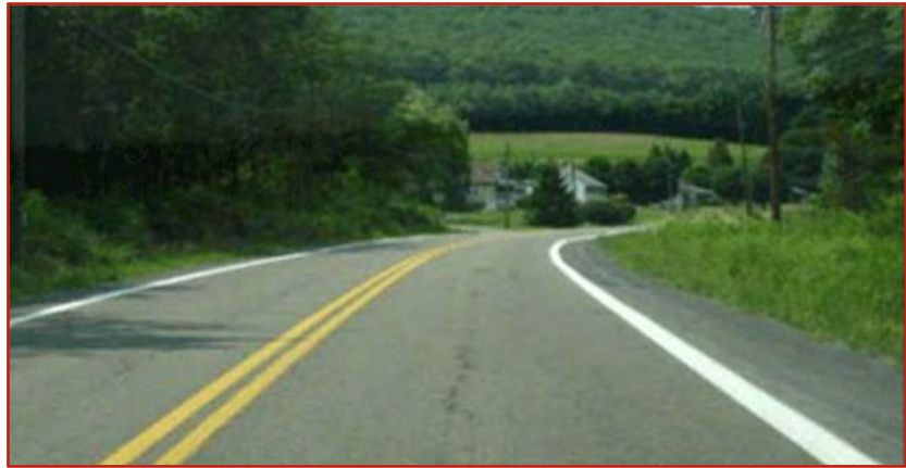
Figure 4-17. Road with Wide, Eight-Inch Pavement Marking Edge Line
