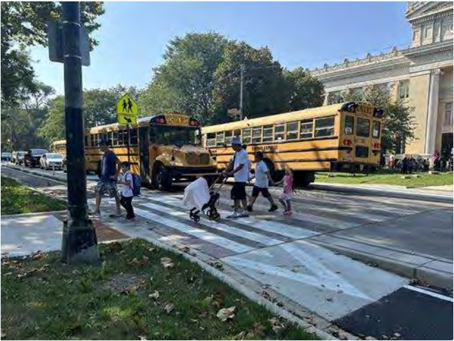
A raised crosswalk across 24th Blvd in front of Saucedo Elementary School provides a safe crossing and increased pedestrian visibility.
