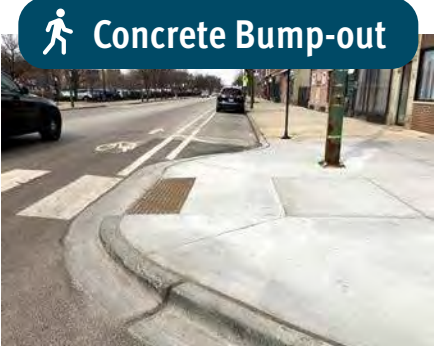
Curb bump-outs and concrete refuge islands reduce crossing distances for pedestrians on Milwaukee Ave and slow motor vehicles.
