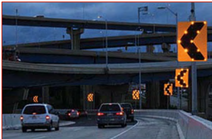
Figure 4-16. Example of Sequentially Flashing LED Chevrons
