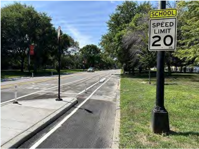
Protected bike lanes and a lower speed limit reduce conflicts between cyclists and motorists as they approach the school.
