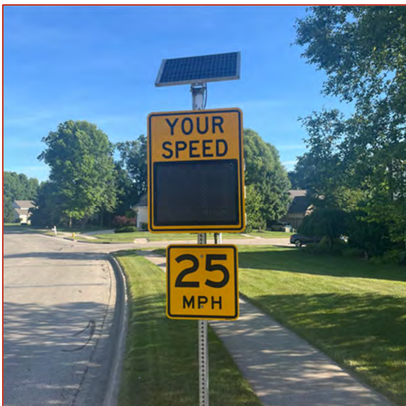
Figure 4-18. Example of Dynamic Speed Feedback Sign on Roadside
