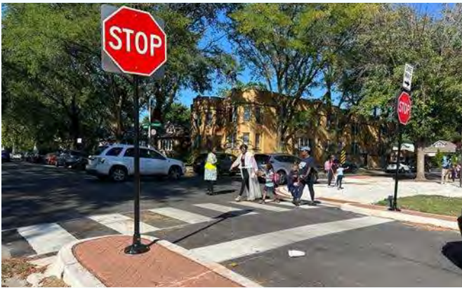
Bump-outs at the corner of 78th St and Calumet Ave at the northeast corner of Ruggles Elementary School.
