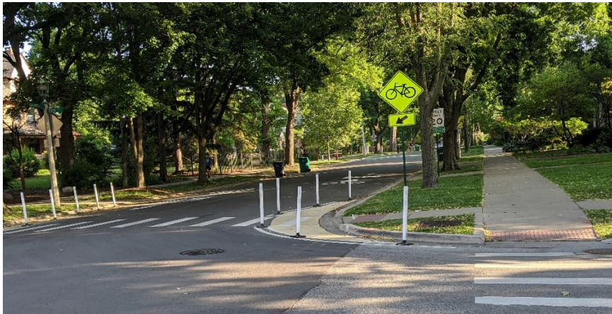
Temporary curb extension in Oak Park, IL
