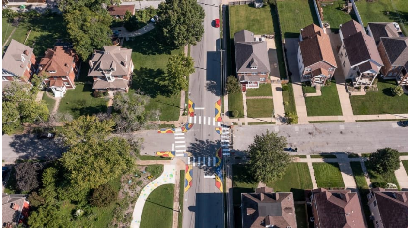
Paint and post intersection in Saint Louis, MO
