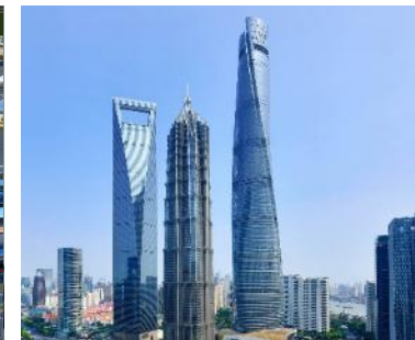
SHANGHAI TOWER Shanghai, China
