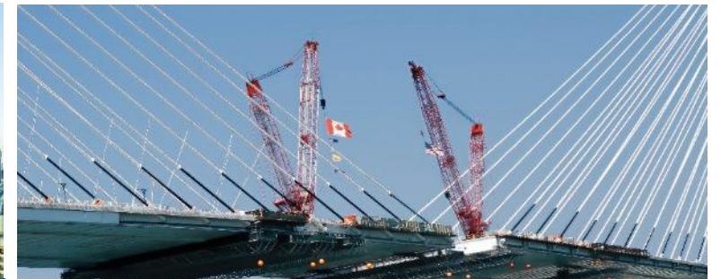
GORDIE HOWE INTERNATIONAL BRIDGE United States and Canada
