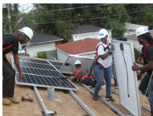
Figures 12 & 13. Workers installing solar panels. Image credit: Elevate.
