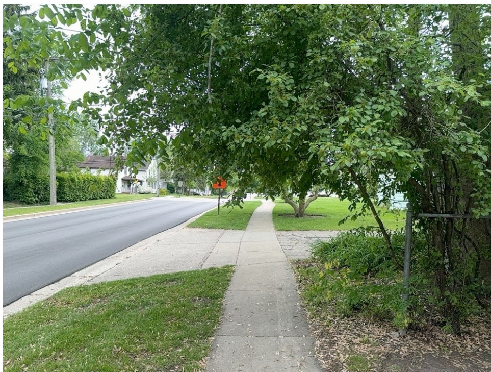
FIGURE 8. EXAMPLE OF SIDEWALK WITH TEMPORARY VEGETATION OBSTRUCTION
