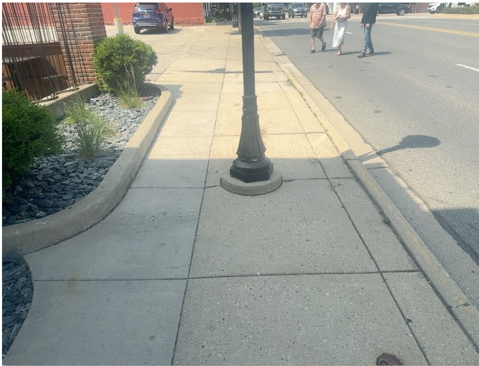
FIGURE 7. EXAMPLE OF SIDEWALK WITH PERMANENT OBSTRUCTION
