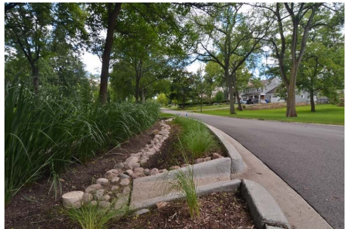
Example of parkway rain garden with curb cuts to capture street runoff. Courtesy of Center for Neighborhood Technology
