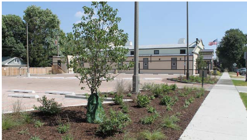
Permeable paver parking lot at Liberty Cultural Center. Photo courtesy of Berwyn Park District.
