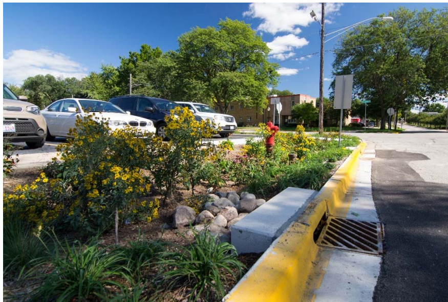
This rain garden captures runoff from the street and adjacent parking lot. Courtesy of Center for Neighborhood Technology.
