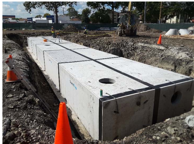
Installation of StormTrap system in Proksa Park.
