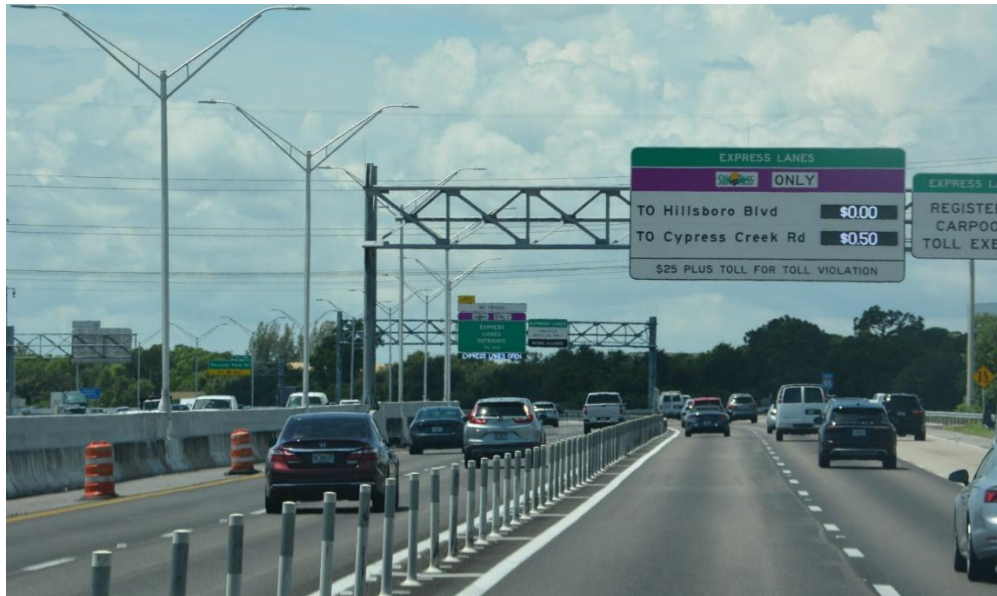
Figure 2. Example of physical separation between tolled and untolled lanes. 8
