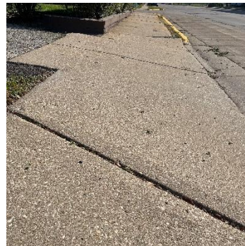
_____ Steep Cross Slope (e.g. sidewalk is not flat)
