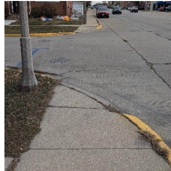
_____ No Detectable Warning Panels (e.g. bumps at the bottom of the curb ramp)
