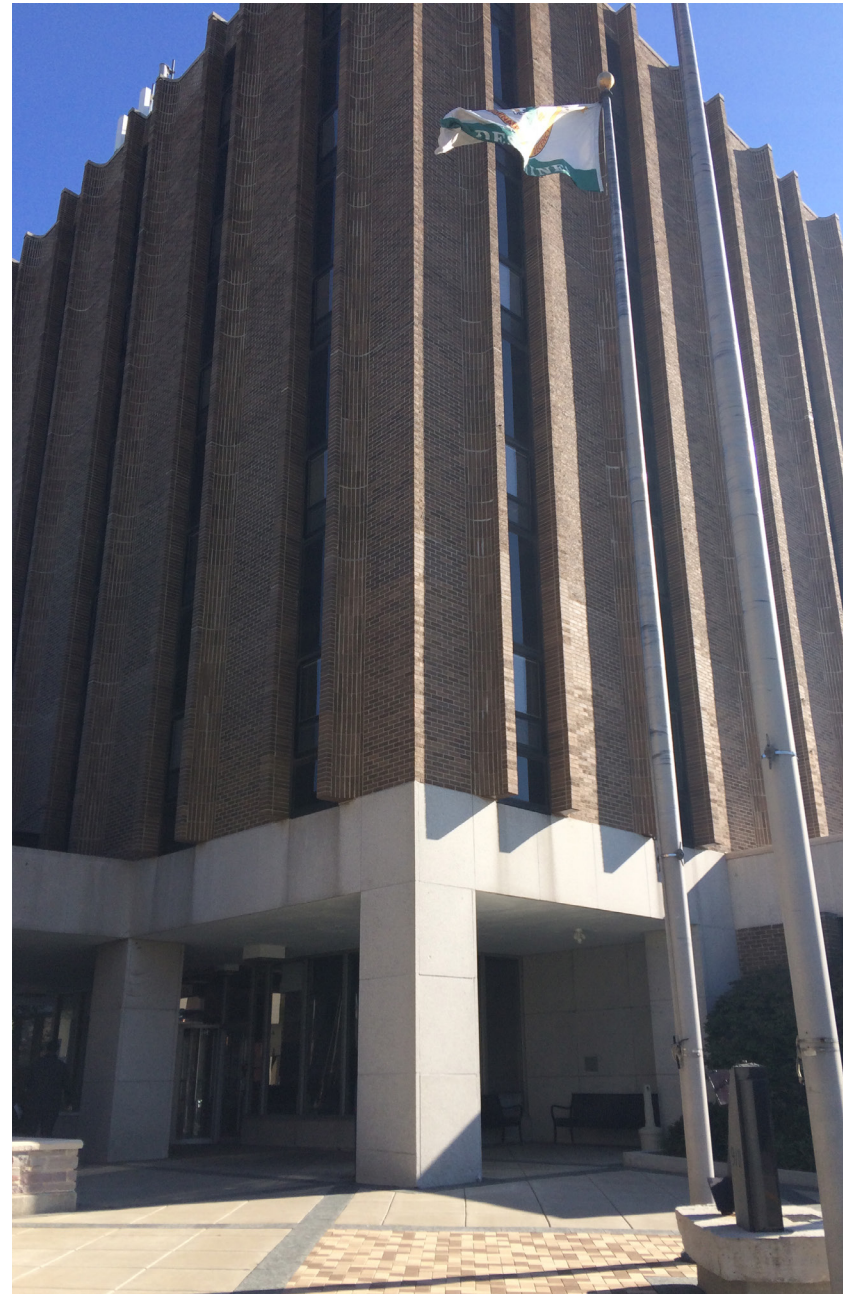
Des Plaines City Hall on Miner Street
