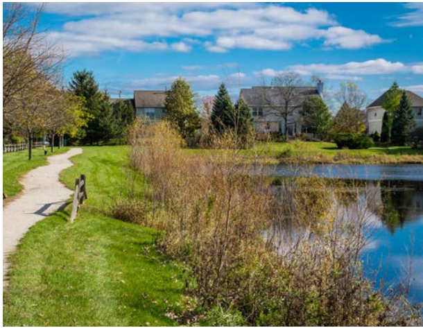
Example of a stormwater detention basin in Port Barrington that incorporates native vegetation and a recreational path.
