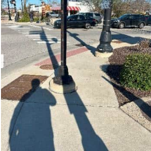
_____ Obstruction (e.g. utility poles, fire hydrants etc.)
