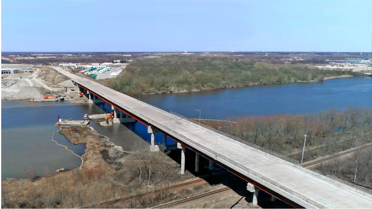
Figure 3: Houbolt Road Bridge Construction 69
