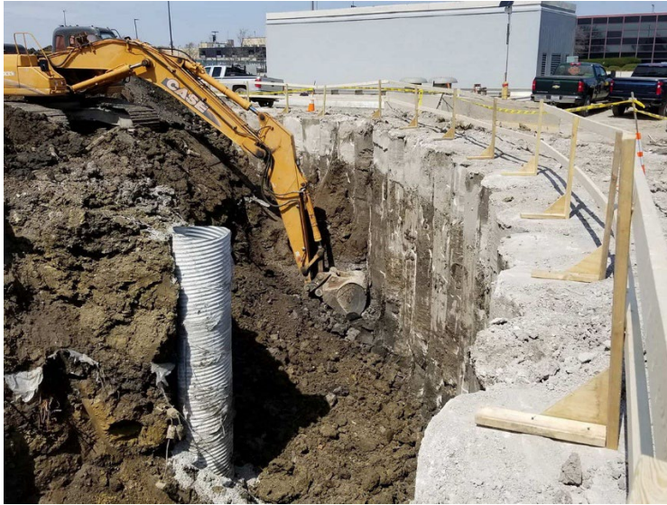
Figure 2: I-290 Pump Station Construction 66
