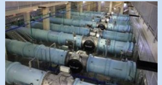
From Top to Bottom: Water Replenishment District in Southern CA; Water Sanitation Area in Cincinnati, OH; Water Treatment Plant in San Diego, CA
