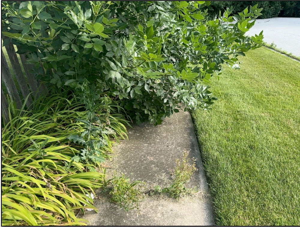
FIGURE 8. TEMPORARY VEGETATION OBSTRUCTIONS
