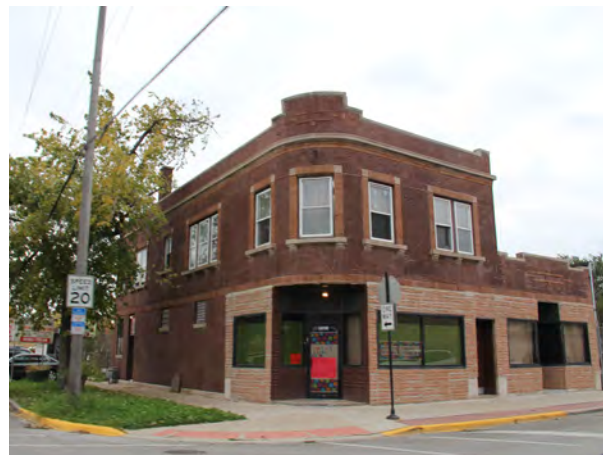
Traditional corner commercial building located within a residential neighborhood.
