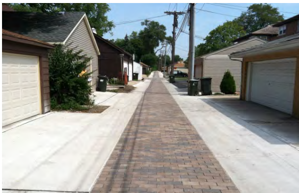
Permeable Paver Application in a Residential Alley Setting.
