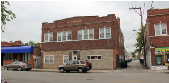
An example of an existing bricked-in storefront in Cicero.
