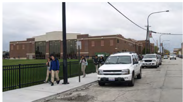
Infrastructure improvements should also be targeted in areas for planned redevelopment, including a proposed Institutional Campus.
