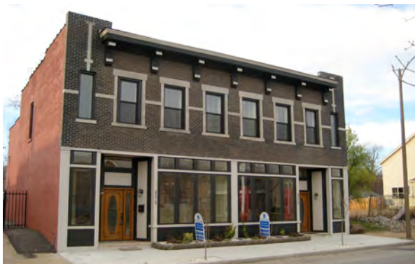
A properly converted storefront residential unit in St. Louis, Missouri. Image courtesy of vanishingstl.blogspot.com .
