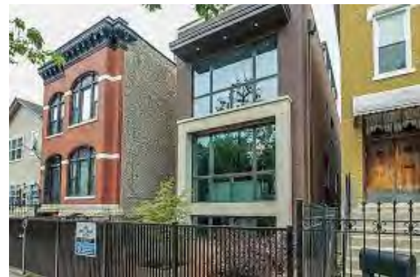
New two-flat infill construction, Chicago.
