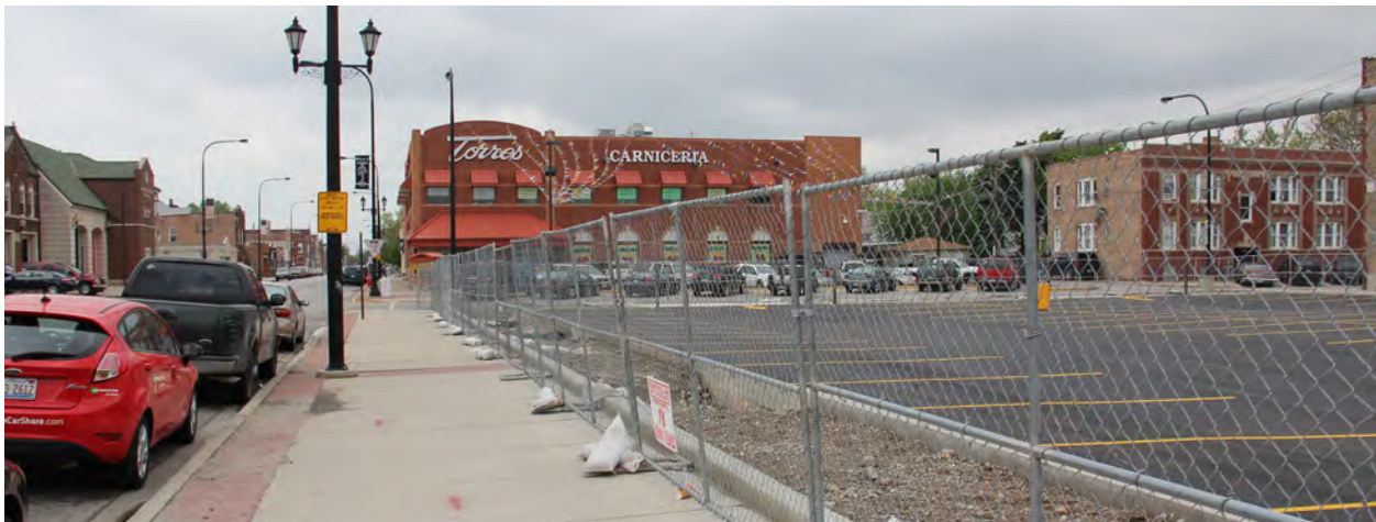
An off-street parking lot under construction on 25th Street.
