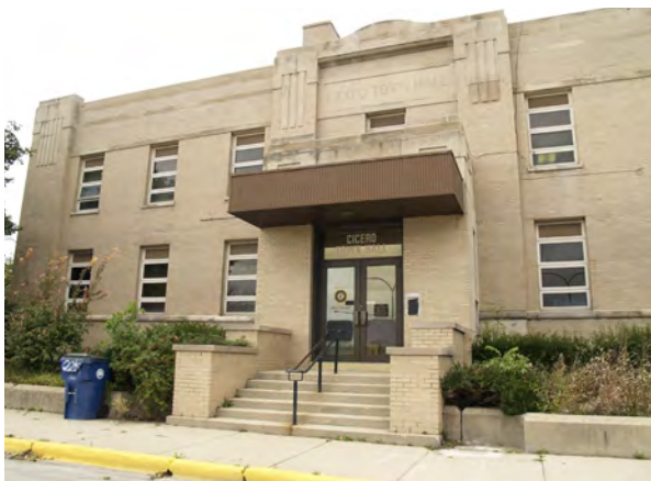
The former Town Hall.
