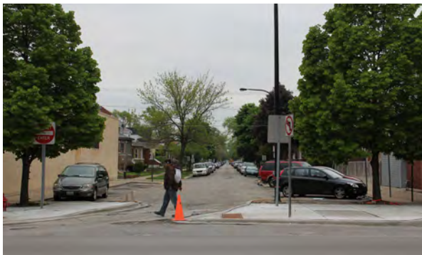
Intersection in need of improvements.
