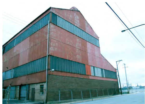
Kropp Forge complex along 54th Avenue.
