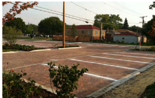
Permeable Paver Application in Business District Parking Lot.
