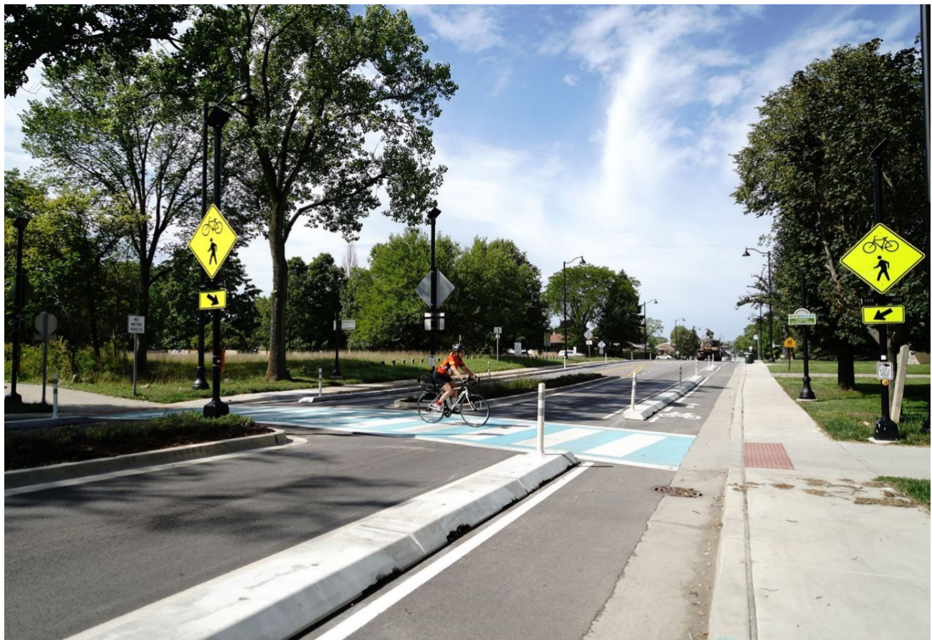
Figure 23. A road diet with a planted median in Niles, Illinois, improved safety by reducing the width of the roadway and slowing vehicle speeds with visual friction
