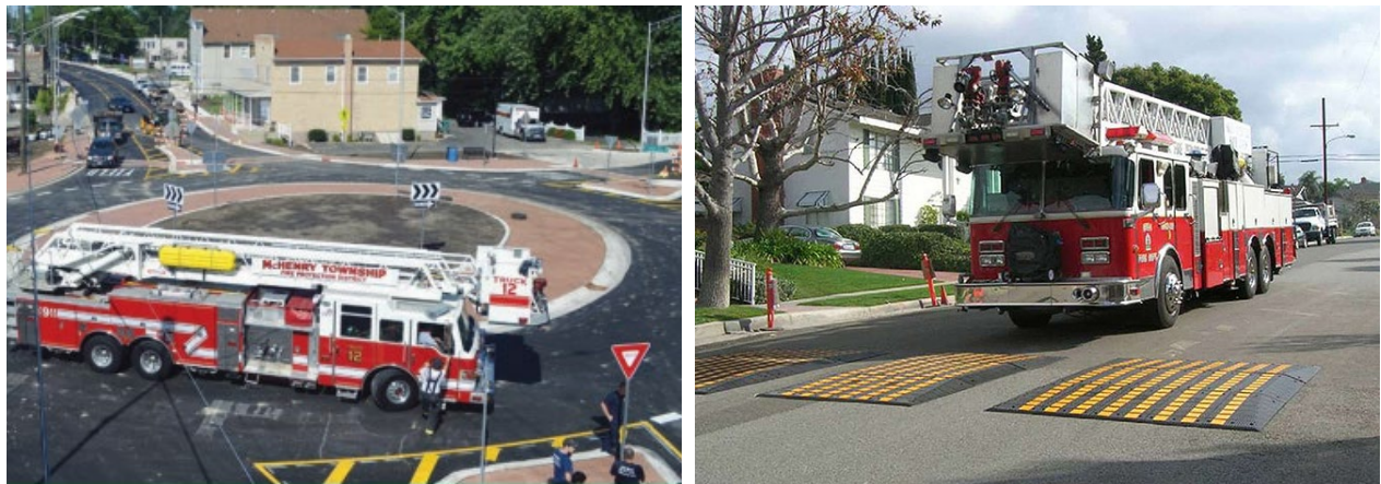
Figure 29. Traffic calming features like mountable aprons (left) and speed hump cutouts, also referred to as speed lumps (right), can be designed to allow emergency access
